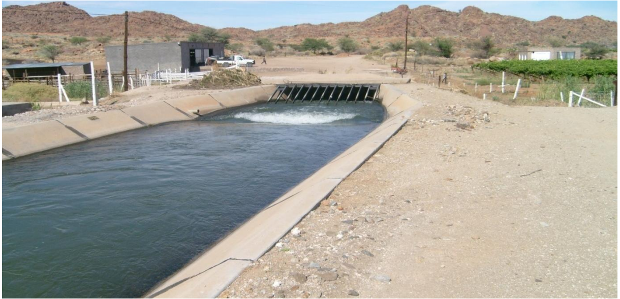
Figure 4-1: Siphon and canal condition
