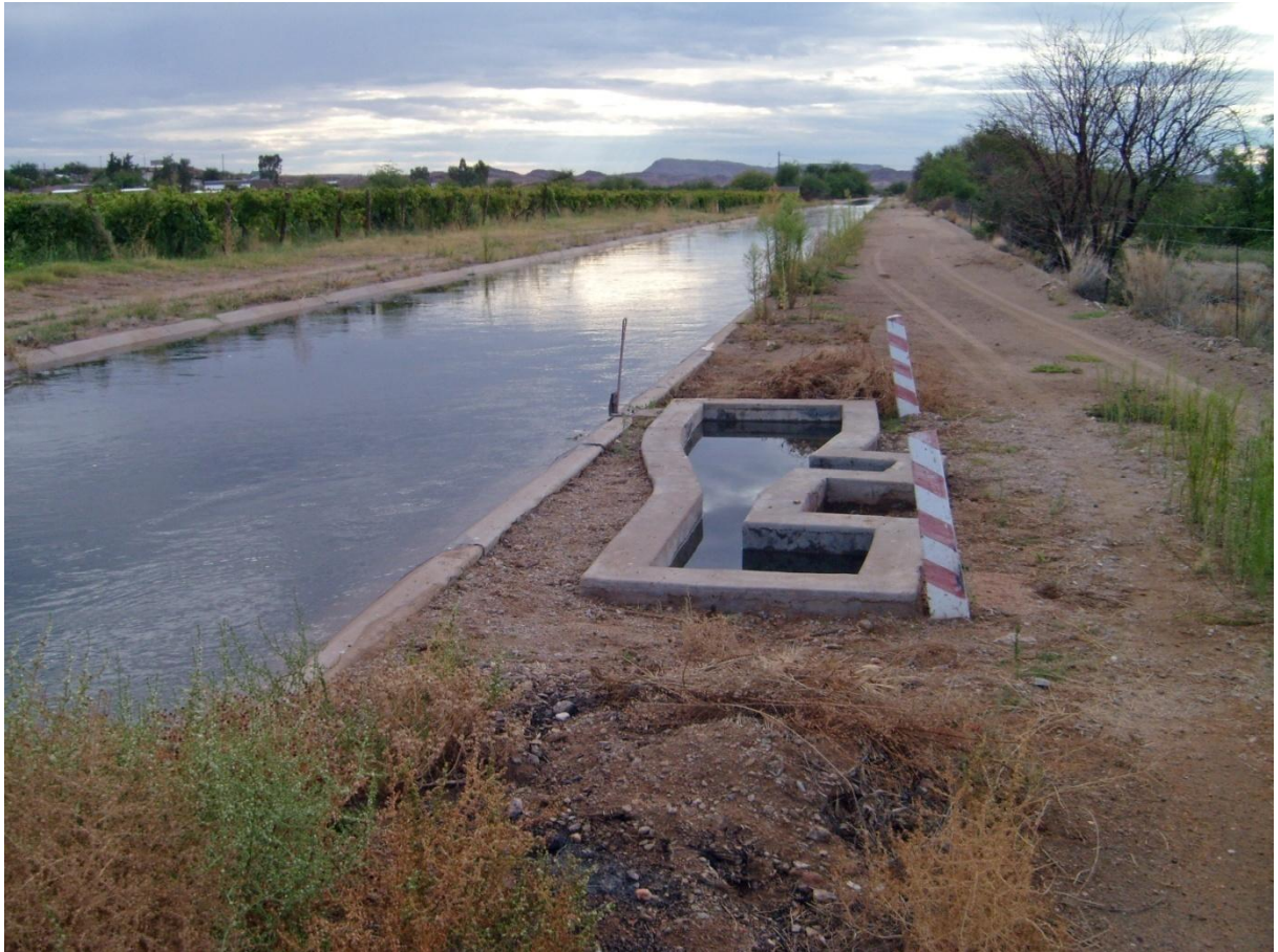
Figure 3-5: User outlet on Northern canal
