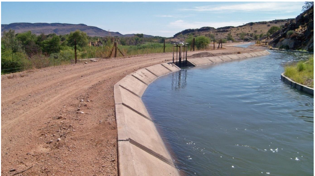
Figure 4-2: Condition of main canal
